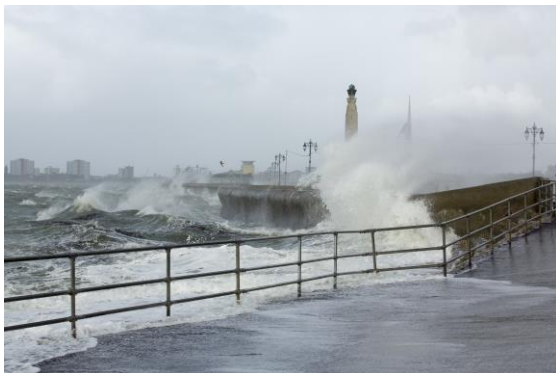
Figure 1. High waves from storm Brian batter Southsea coastal path, UK, October 2017
